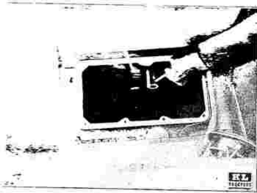
Fig. 51. Unscrewing big end nuts.
